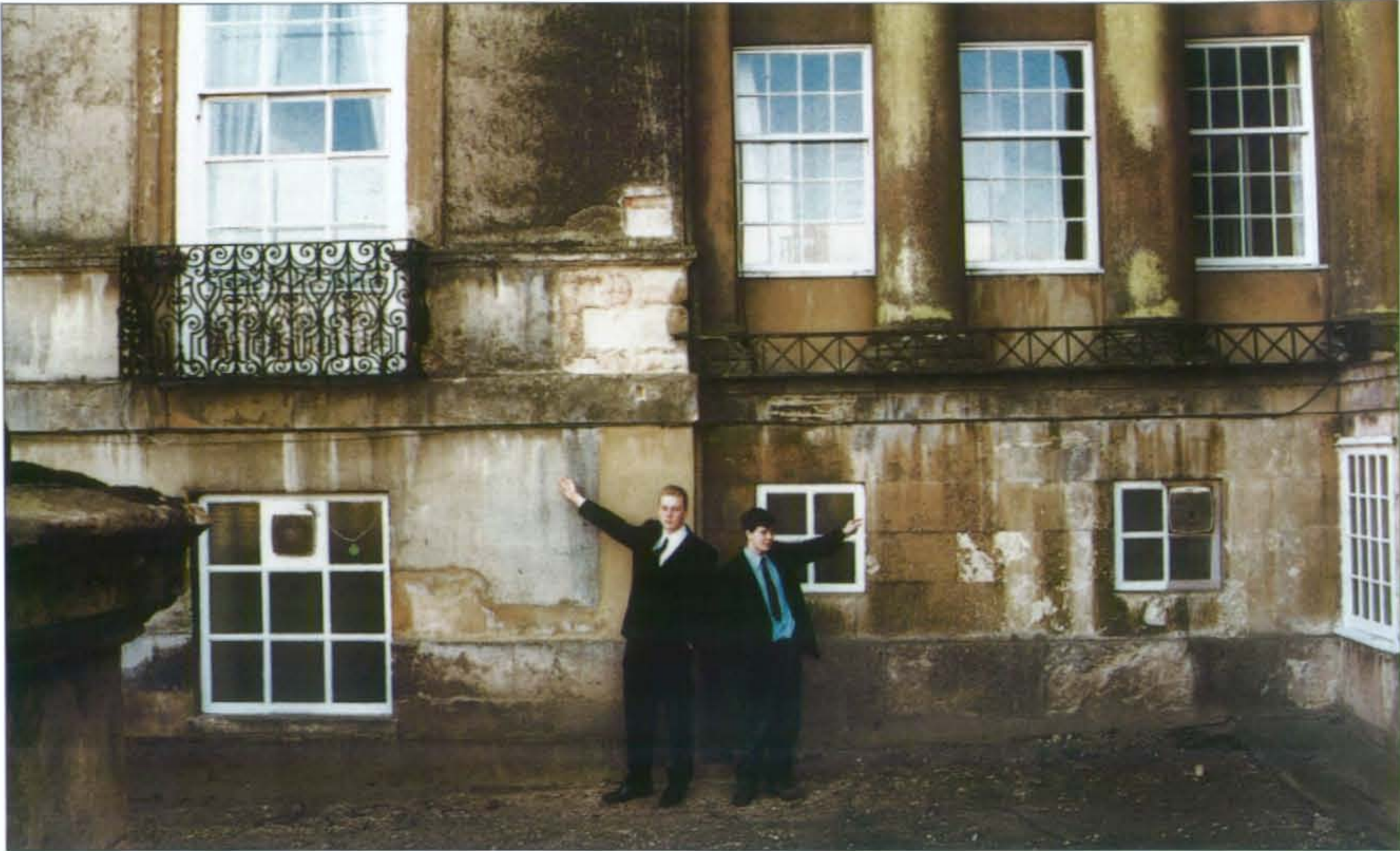
Where the later colonnades meet the earlier mansion: Duncan (left) points to the stuccoed base of the mansion. Charles (right) points to the ashlar of the podium of the colonnades. The rooms between the columns are nineteenth-century infill.
