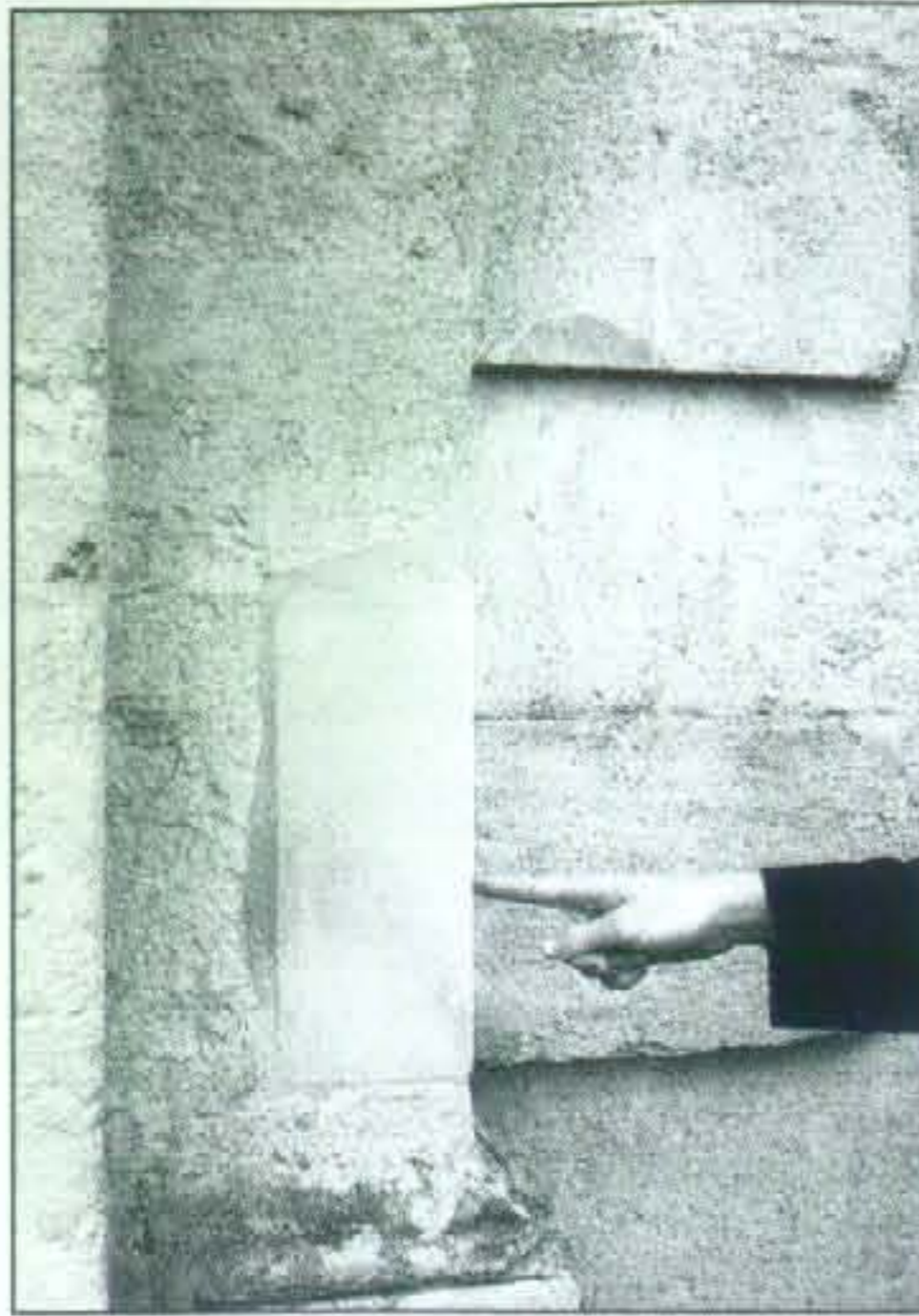
The two different kinds of restoration of stone in a Leoni Arch. In one case a completely new stone has been put in. In the other the weather-worn part has been protected by some form of rendering.
