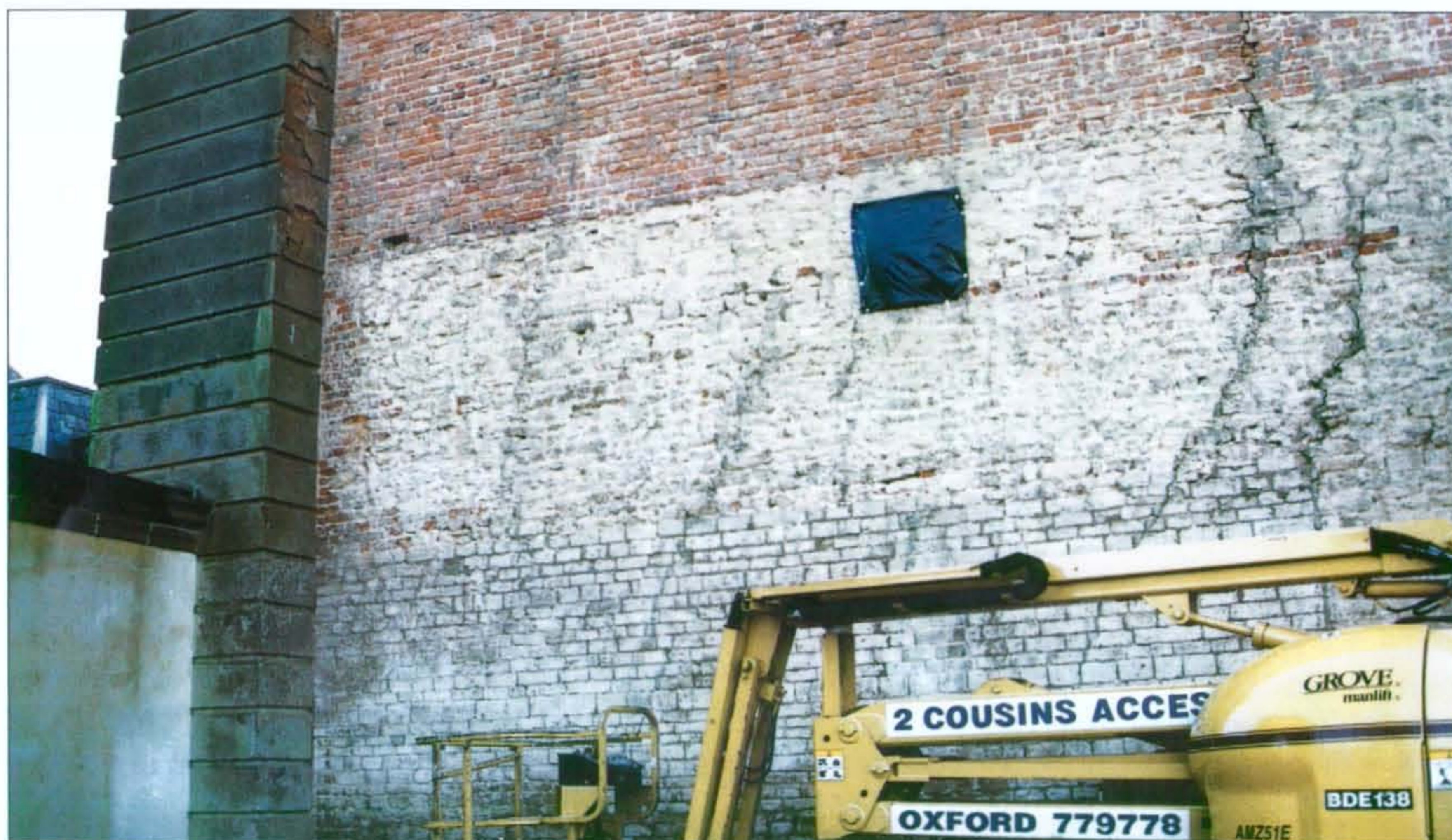
January 2000: Exploratory work on the screen wall between the Grafton Arch and the entrance to Cobham Court revealed three distinct levels of brickwork underneath the stucco covering
