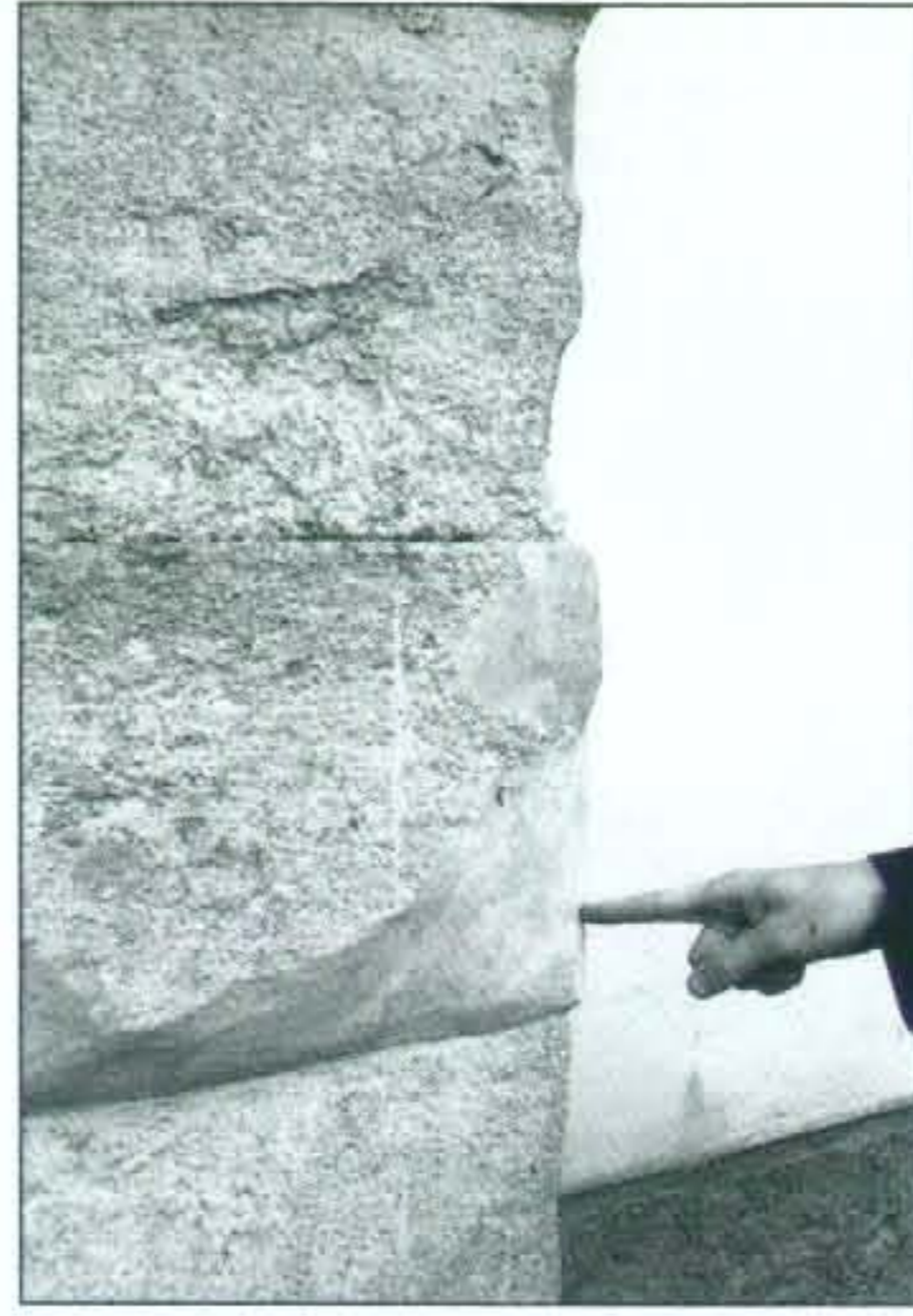
The two different kinds of restoration of stone in a Leoni Arch. In one case a completely new stone has been put in. In the other the weather-worn part has been protected by some form of rendering.
